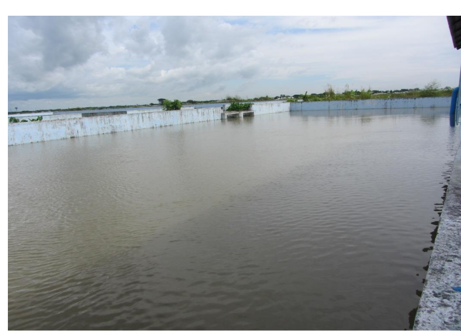
Pre-sedimentation Basin and Low Lift Pump for Aeration and Create Overflow Weir
