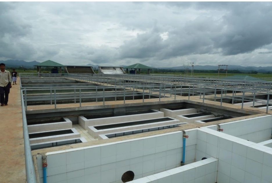
Pre-sedimentation Basin and Low Lift Pump for Aeration and Create Overflow Weir
