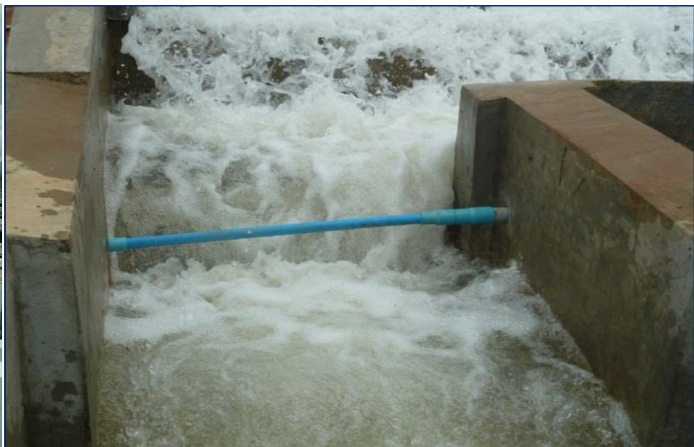
Pre-sedimentation Basin and Low Lift Pump for Aeration and Create Overflow Weir
