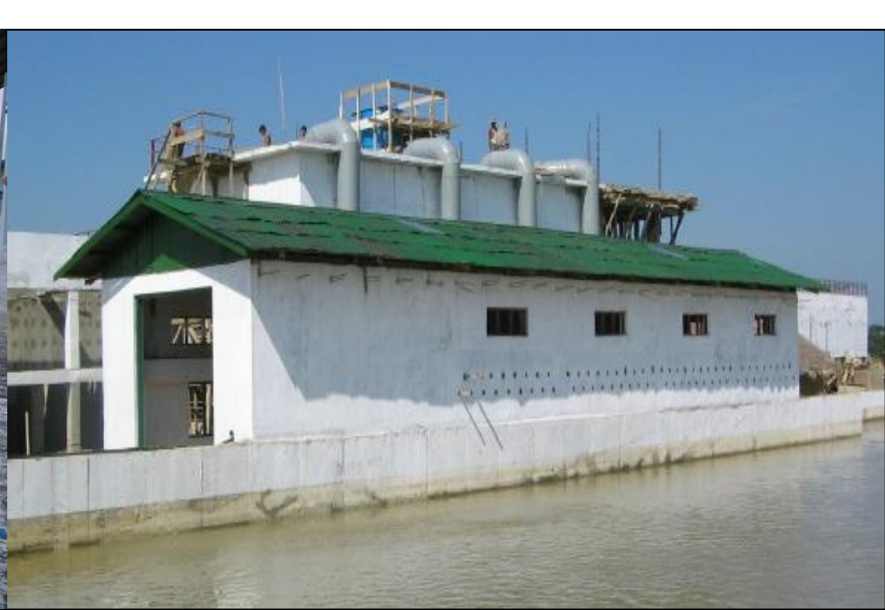
Pre-sedimentation Basin and Low Lift Pump for Aeration and Create Overflow Weir
